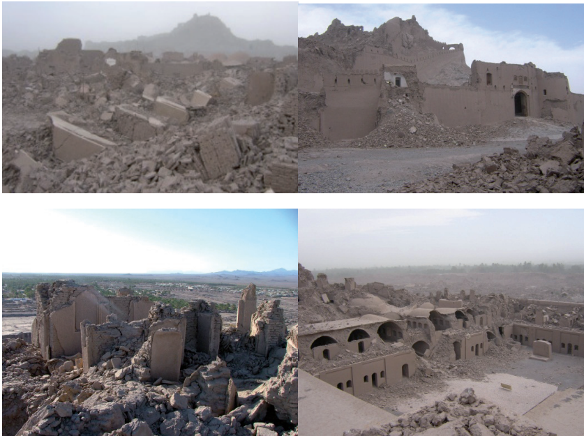
Figure 1. Citadel of Bam after earthquake in 2003
