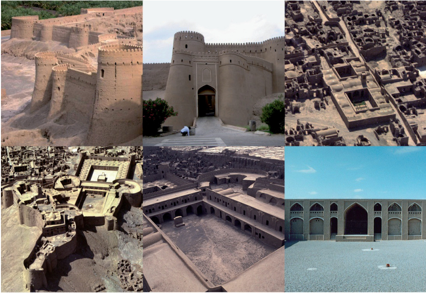
Figure 2. Architecture of citadel of Bam and its different types of buildings. Photographic credits: ICHHTO (top left, center, bottom center, and right) and NCC (top right and bottom left)
